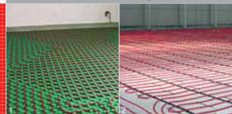
1 ► Installation with preformed panel
