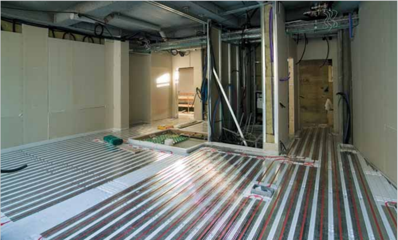
installation of underfloor system
