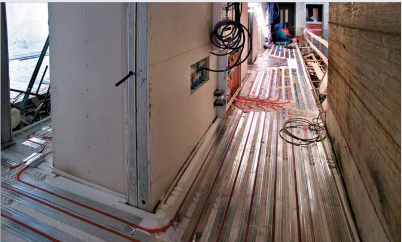
detail of distribution, starting from manifold R559
